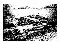
(b) via a sand carrier whereby sand is loaded onto the sand carrier and discharged directly onto the dumping site via a conveyor belt system.
